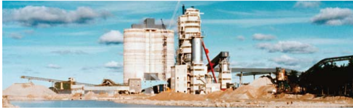
Many of Nordkalk's customers depend on the excellent quality of Gotland limestone. Stone from Storugns is burned into quicklime e.g. in the kiln of KPAB.
