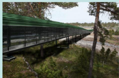
as possible, an 8.7-km-long conveyor belt will be built from Bunge to Storugns. The belt will mostly be covered, which will reduce both noise and dust emissions. It will also be raised to permit free passage by people and wildlife alike.
